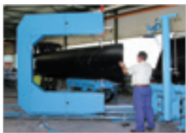
Mitre cutting a 1000 mm diameter pipe
